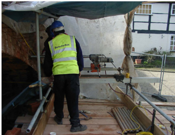
Fig. 2. Drilling the transverse holes in the arch barrel.
