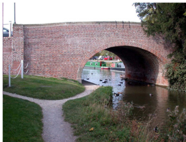
Fig. 5. A view of the successfully strengthened bridge.
