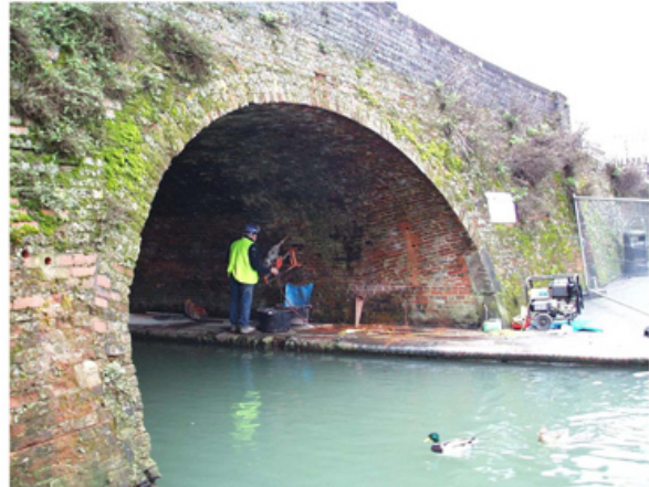
Fig. 4. Drilling the holes for the radial inter-ring dowels.
