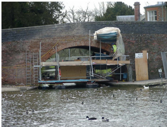
Fig. 1. Hungerford Canal Bridge showing the pontoons and working platform.
