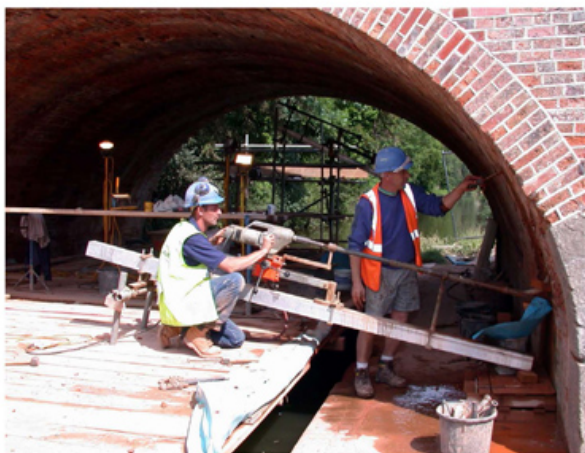
Fig. 3. Drilling the holes for the longitudinal reinforcement.
