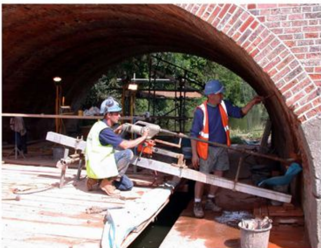
Fig. 3. Drilling the holes for the longitudinal reinforcement.
